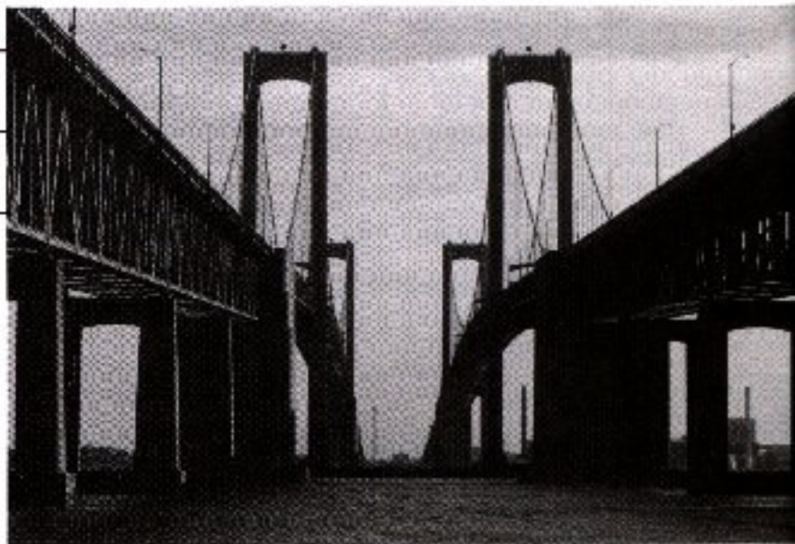
Delaware Memorial Bridge, Wilmington, Delaware
