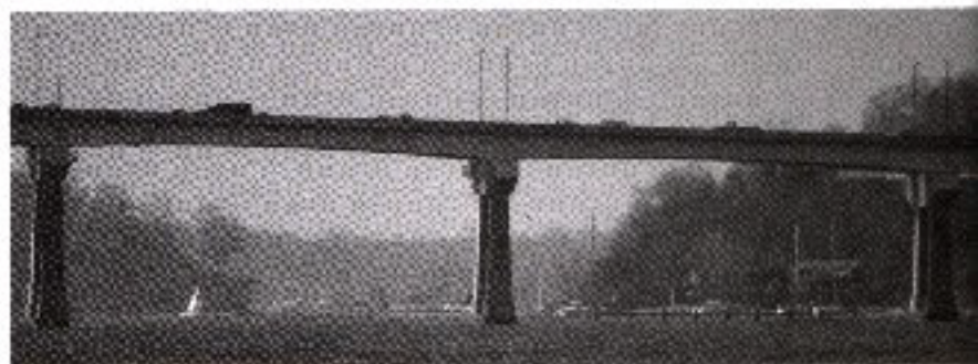
Severn River Bridge, Annapolis, Maryland
