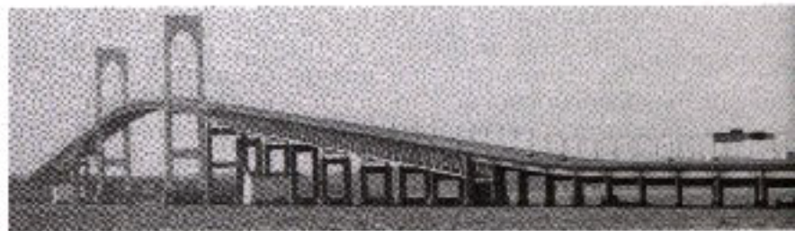
Newport, Rhode Island Bridge
